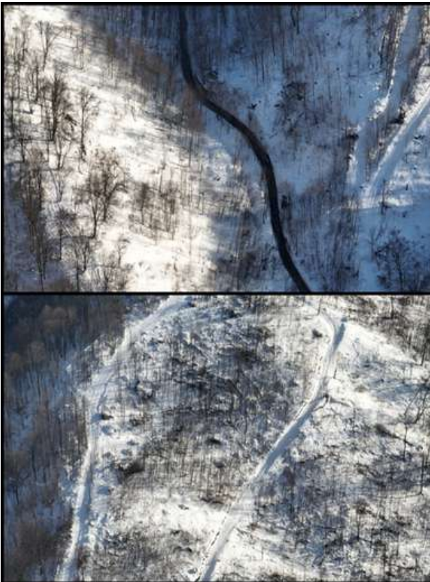
Figure 45: photos illustrating several eroded logging roads, some still in use. Both photos were taken in February 2023.
