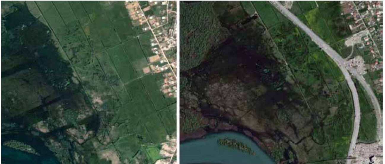
Fig. 4: Construction of new flood dikes in Shkodra (Albania) at the southern end of Skadar Lake will exclude large wetland areas from regular flooding.
