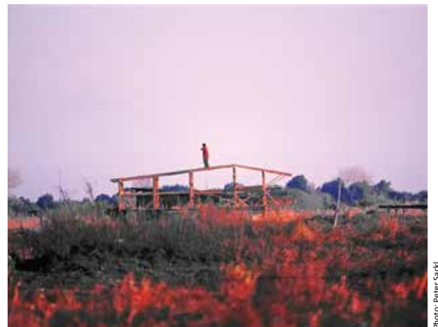
Fig. 5: Construction of a new seaside restaurant in the sand dunes of Velika Plaža, Montenegro, amidst prime nesting habitat of Eurasian Thick-knee and Collared Pratincole, 16 November 2006.
