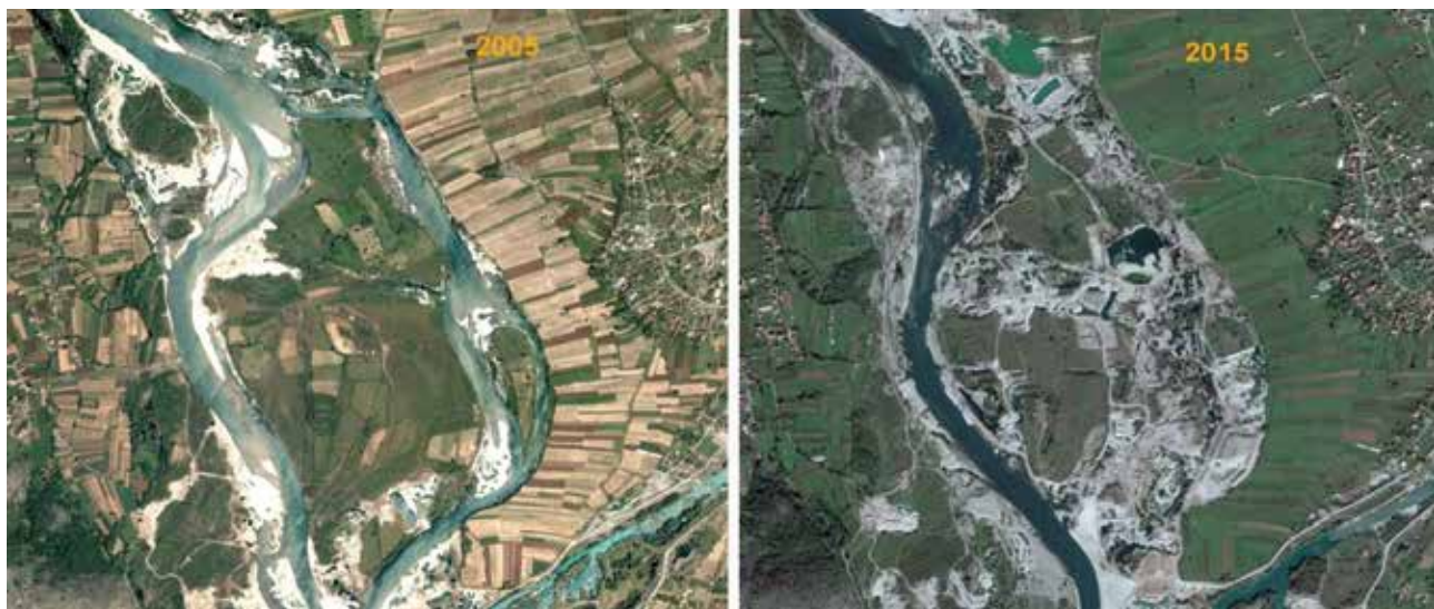
Fig. 7: Destruction of natural riverine habitats through the exploitation of gravel along the lower Morača River in Montenegro just before the river enters Skadar Lake National Park. The ‘moon landscape’ shown in the pictures seems to be the source of construction materials for the entire Podgorica capital region (Google Earth 2019).
