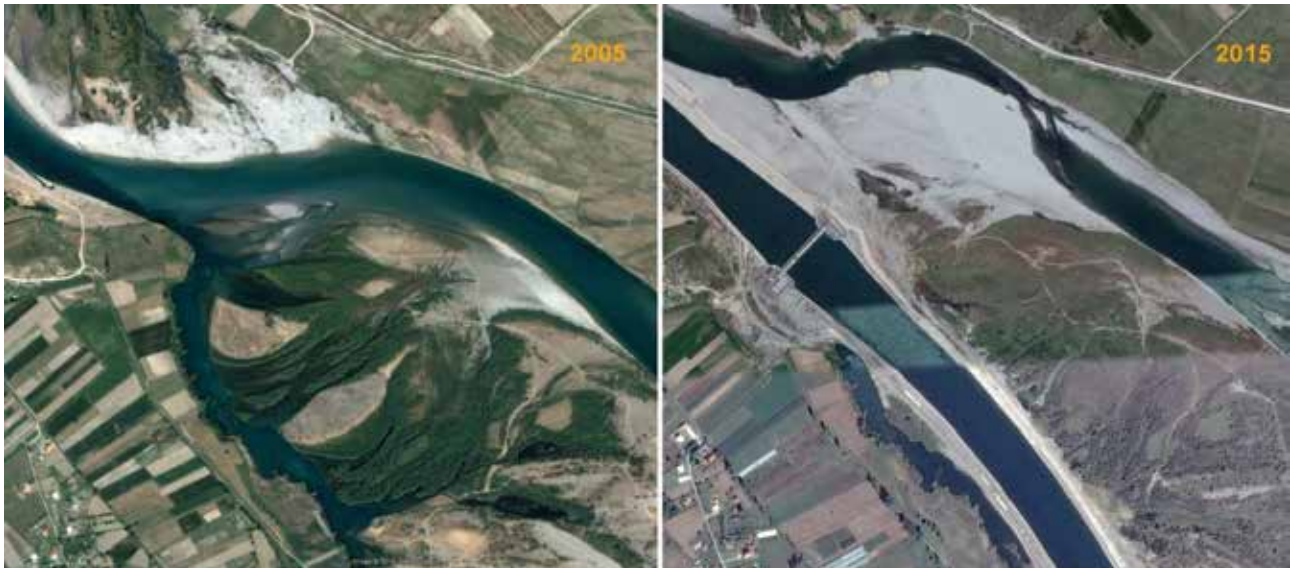
Fig. 5: Construction of two hydropower plants with the abstraction of water through a canal and the remaining stretch of residual water on the lower Drin (Ashta I and II). Up to 90% of water that now flows through the sealed concrete canal, is not available for the natural river system and its floodplain. Consequently, the extent and quality of typical riparian habitats was drastically reduced (Google Earth 2019).
